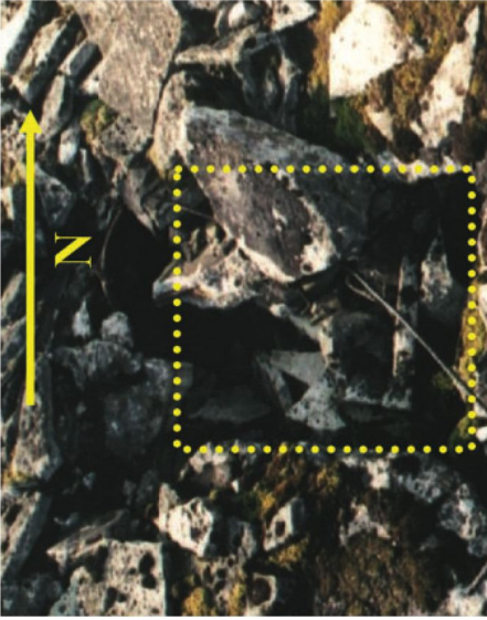
Figure 12. Second (from south) Zykion hole, east to west view. Chunk of concrete torn away by explosion lies atop northern edge; western edge completely shattered. Outline of hole superimposed.
