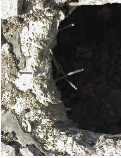
Figure 10c. Close-up view of southern edge of Crematorium III gas chamber, showing the brick wall and the hole. A white arrow points to the hole, and a black arrow points to the 'roof's south-western corner'. The text 'roof's south-western corner' is written in black at the bottom of the image.
