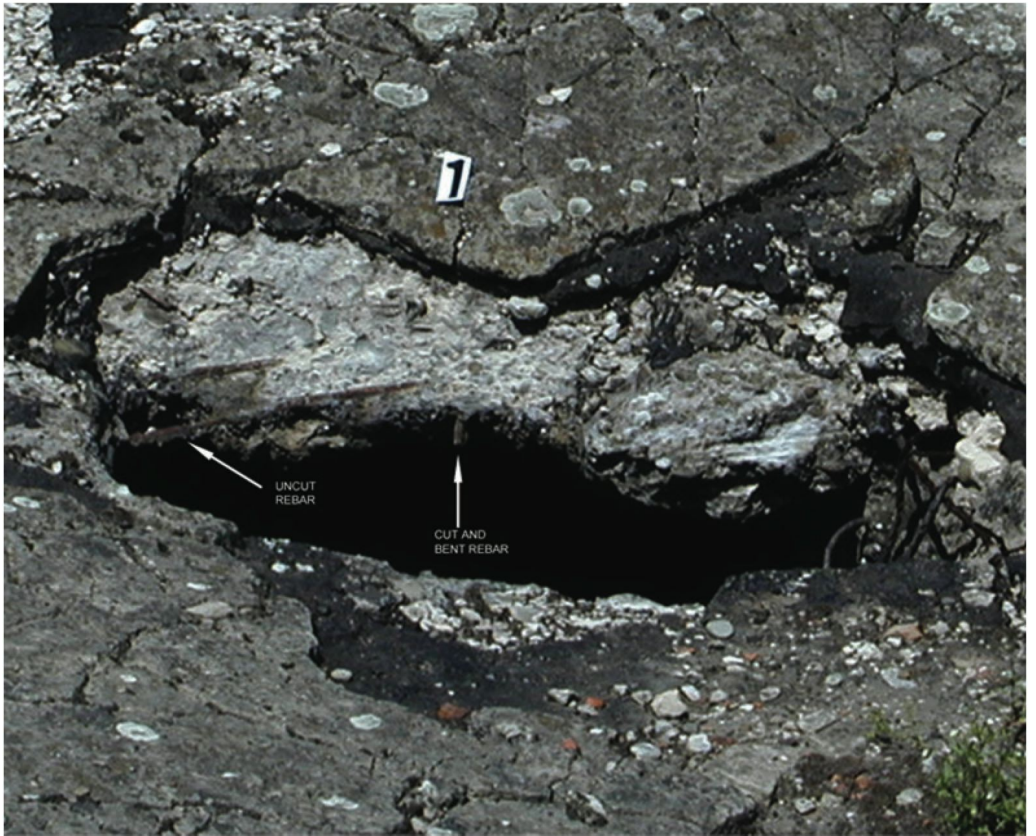
Figure 8b. Area of Zyklon Hole 1, Crematorium II. Tarpaper separating concrete layer below and sand-cement layer above is visible. South to north view.
